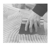
Suitable for bonding of all types of wooden floors such as solid, stab, pre-finished, and on-end parquet, wood-plank, wood-block and laminates.
